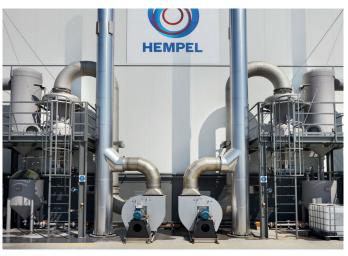
Change over dampers were installed to the flue ductwork to feed an extraction system included two grade 316 lined 13m high chimneys including exhaust gas fans. This system to be on standby in case of failure of third-party installed filtration scrubbers.
